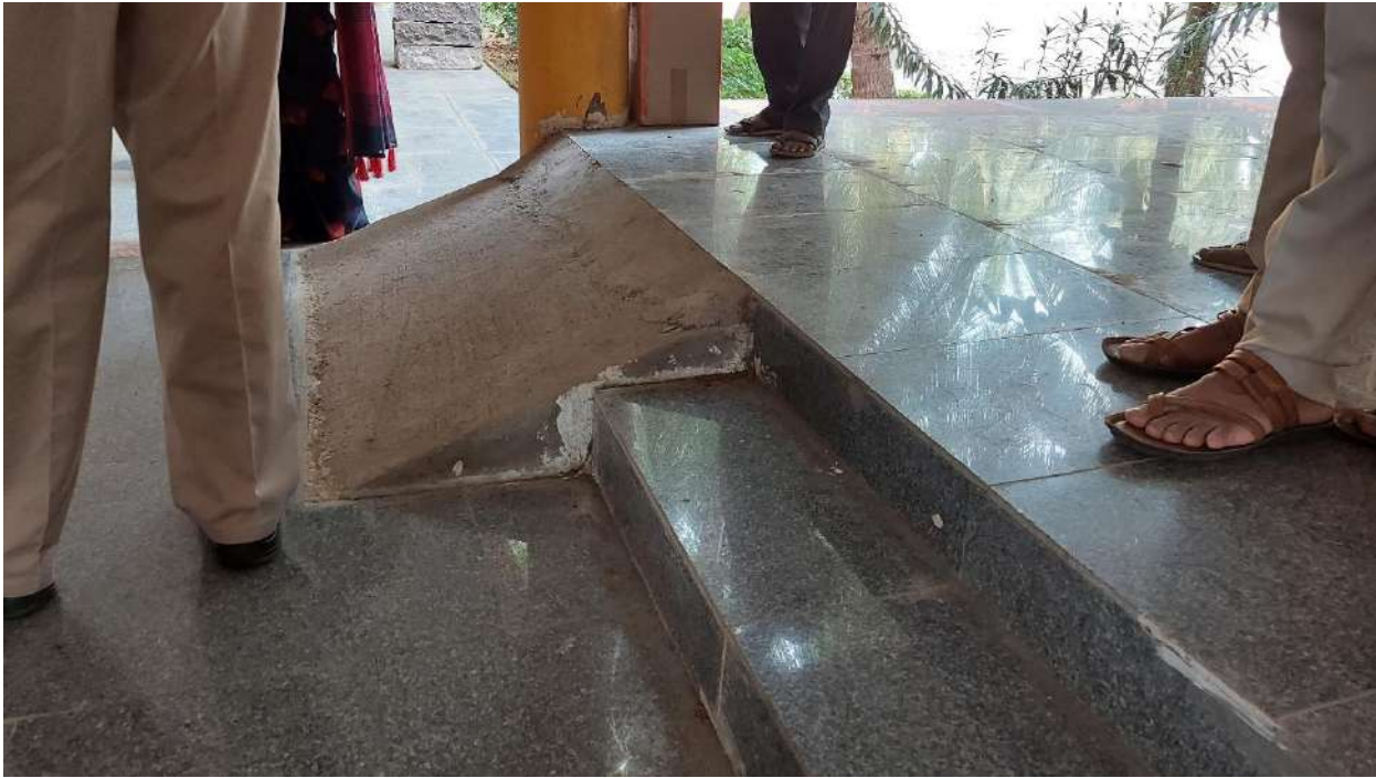
Figure 10 - Placing of ramp for use by physically challenged
