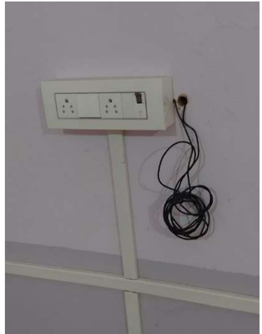
Figure 9 - Loose wiring
