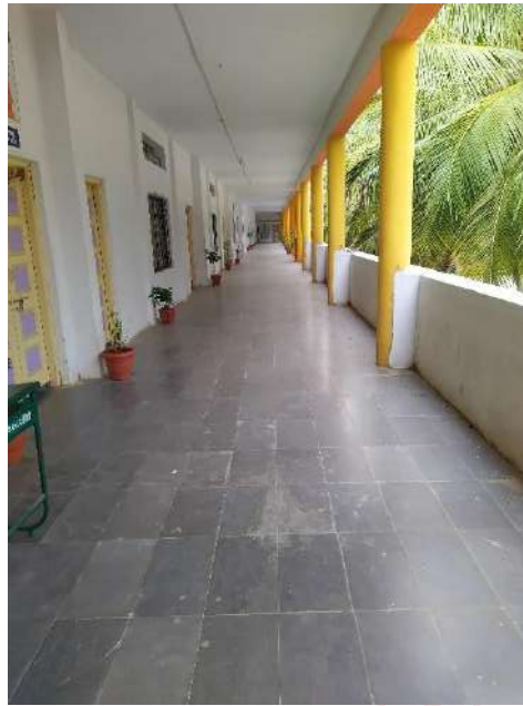
Figure 9 - Missing waste collection bins in the corridor
