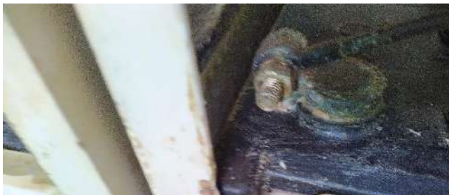
Figure 16 - Galvanic reaction.
