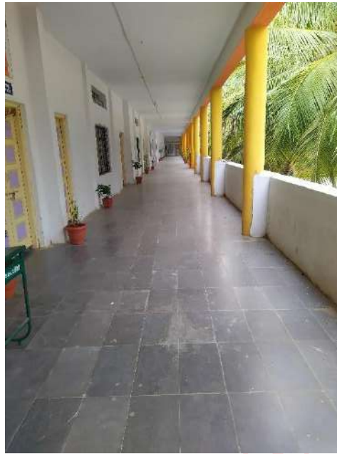
Figure 9 - Missing waste collection bins in the corridor
