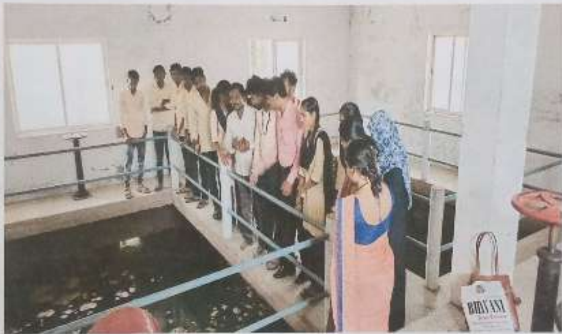
Sand filtration bed
